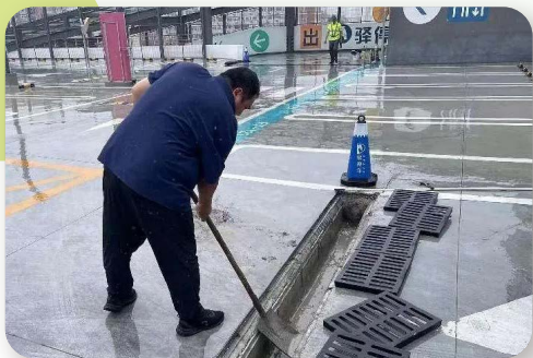
Clearing drainage channels 清除排水通道
