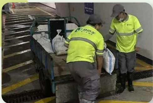
Flood prevention with sandbags 沙袋防洪
